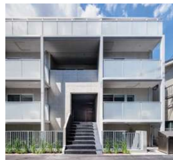
LOGGIA SHIROKANE LOCATION Shirokane, Minato-ku, Tokyo COMPLETION SPECS FLOOR AREA Aug.2024 RC/4F 562㎡
