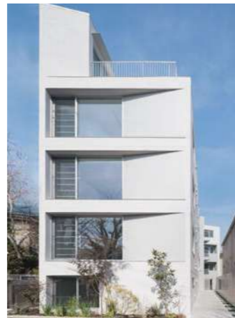
REMBRAN AKATSUTSUMI LOCATION Akatsutsumi, Setagaya-ku, Tokyo COMPLETION SPECS FLOOR AREA Feb.2024 RC/4F 718㎡
