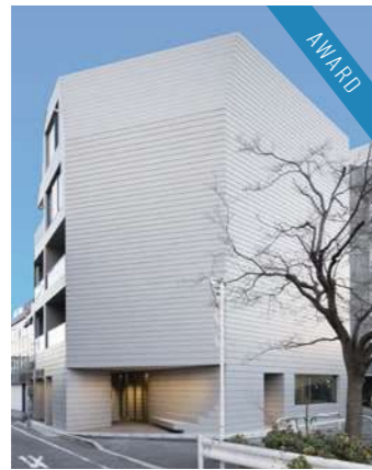
GOOD DESIGN AWARD THE CON-TOUR HATANODAI LOCATION Kamiikedai, Ota-ku, Tokyo COMPLETION SPECS FLOOR AREA Jan.2024 RC/5F 633㎡
