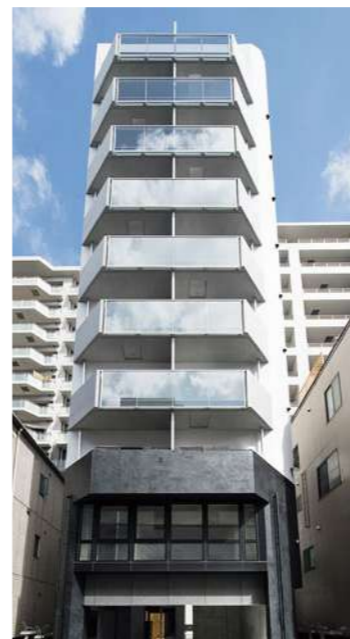
GRAN CASA MONZENAKACHO LOCATION Eitai, Koto-ku, Tokyo COMPLETION SPECS FLOOR AREA Jun.2021 RC/11F 806㎡
